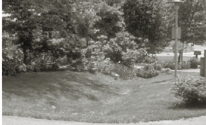
Figure 2-14. Vegetated swale
